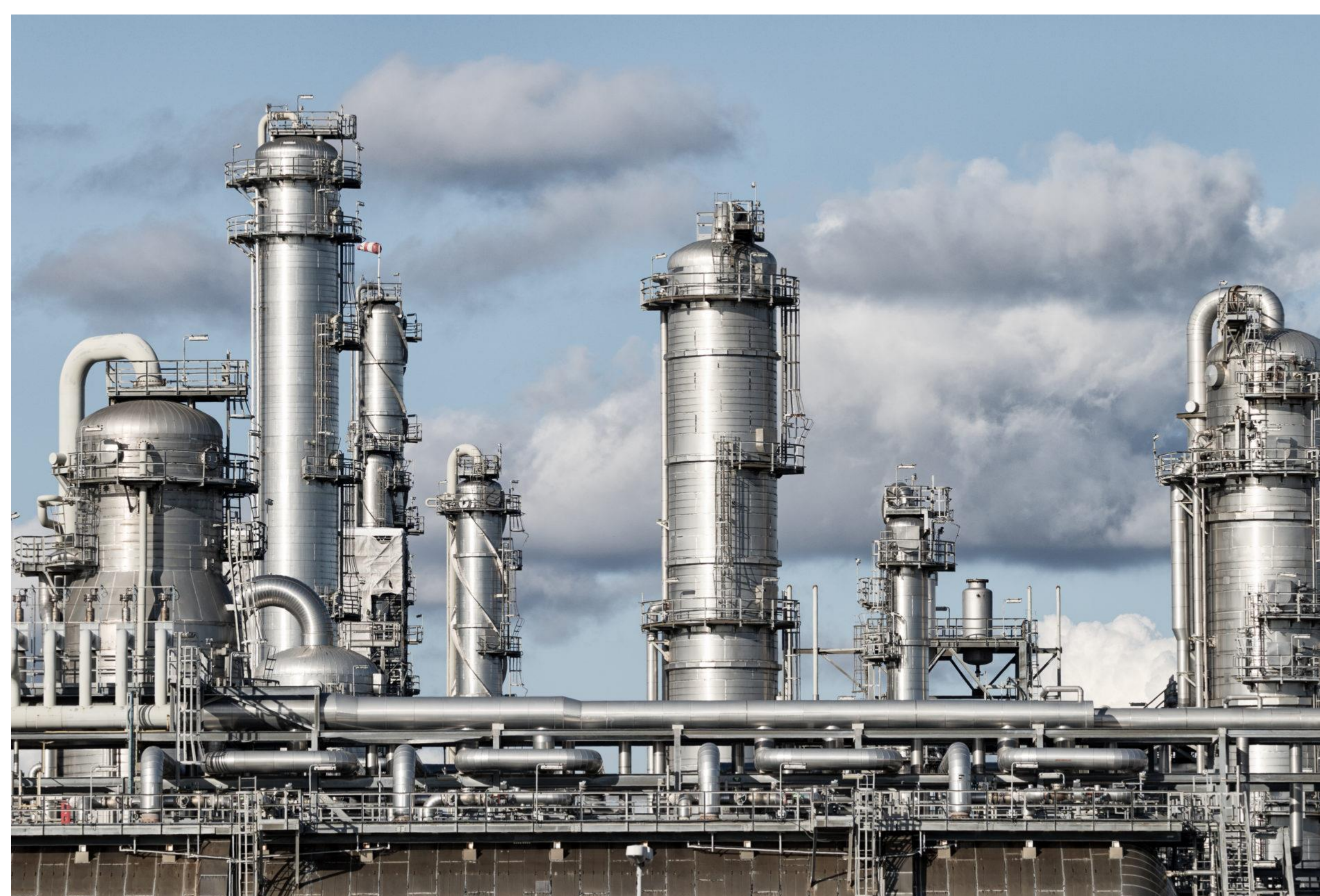
Figure 3. Crude Oil Refinery
