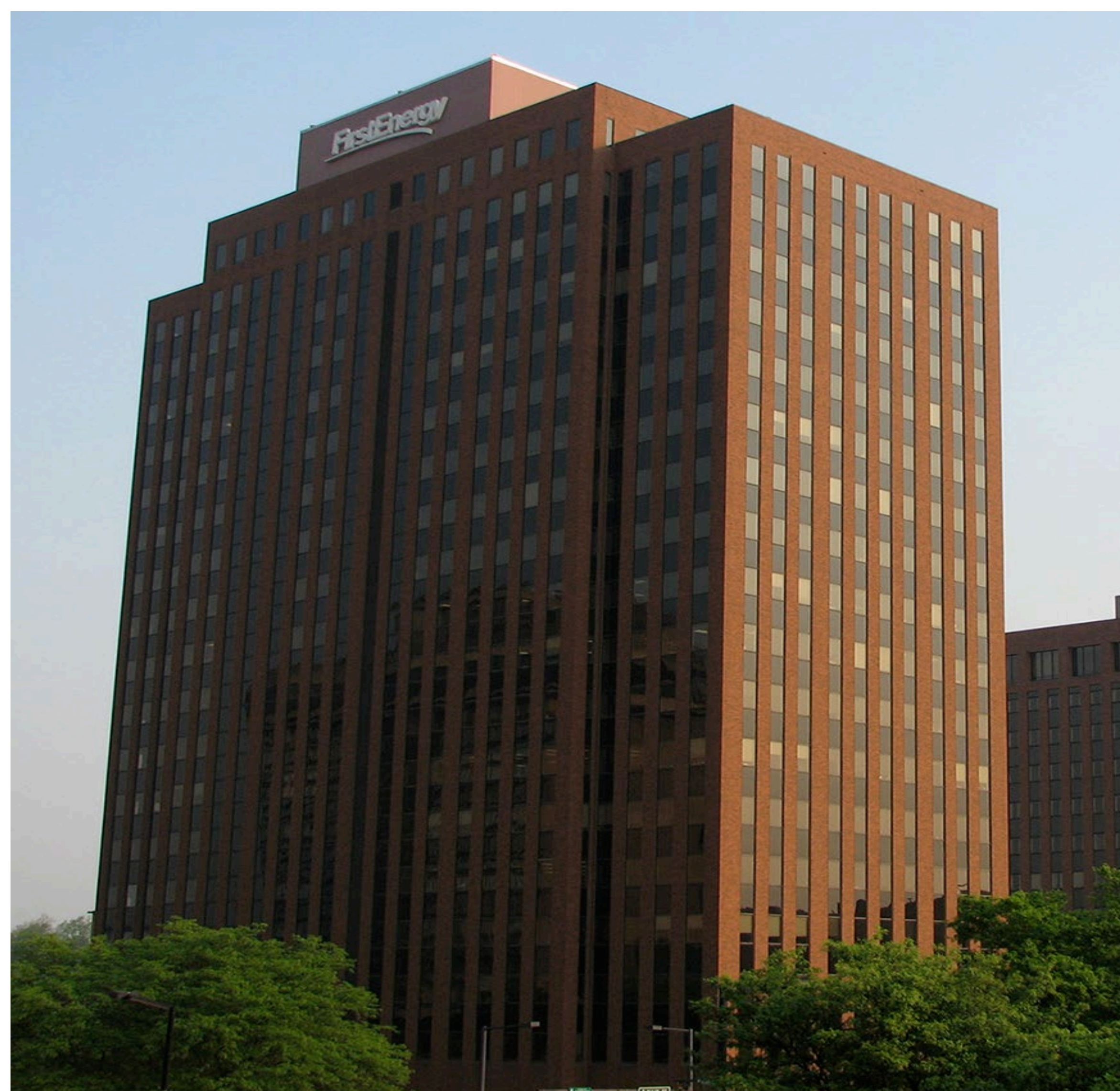
Figure 1. FirstEnergy Headquarters in Akron, Ohio
