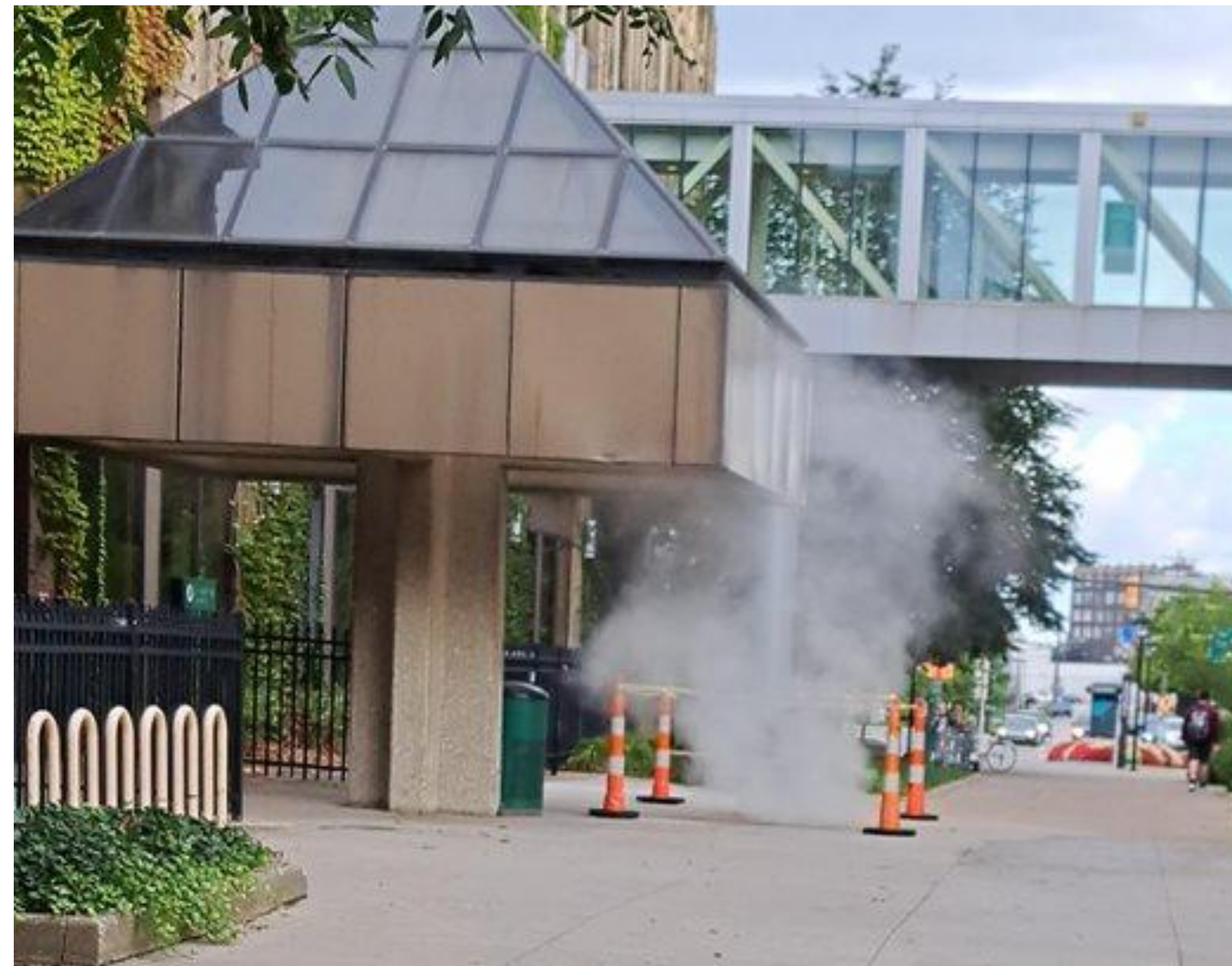
Figure 2. Steam spewing out of the manhole cover on E24th
