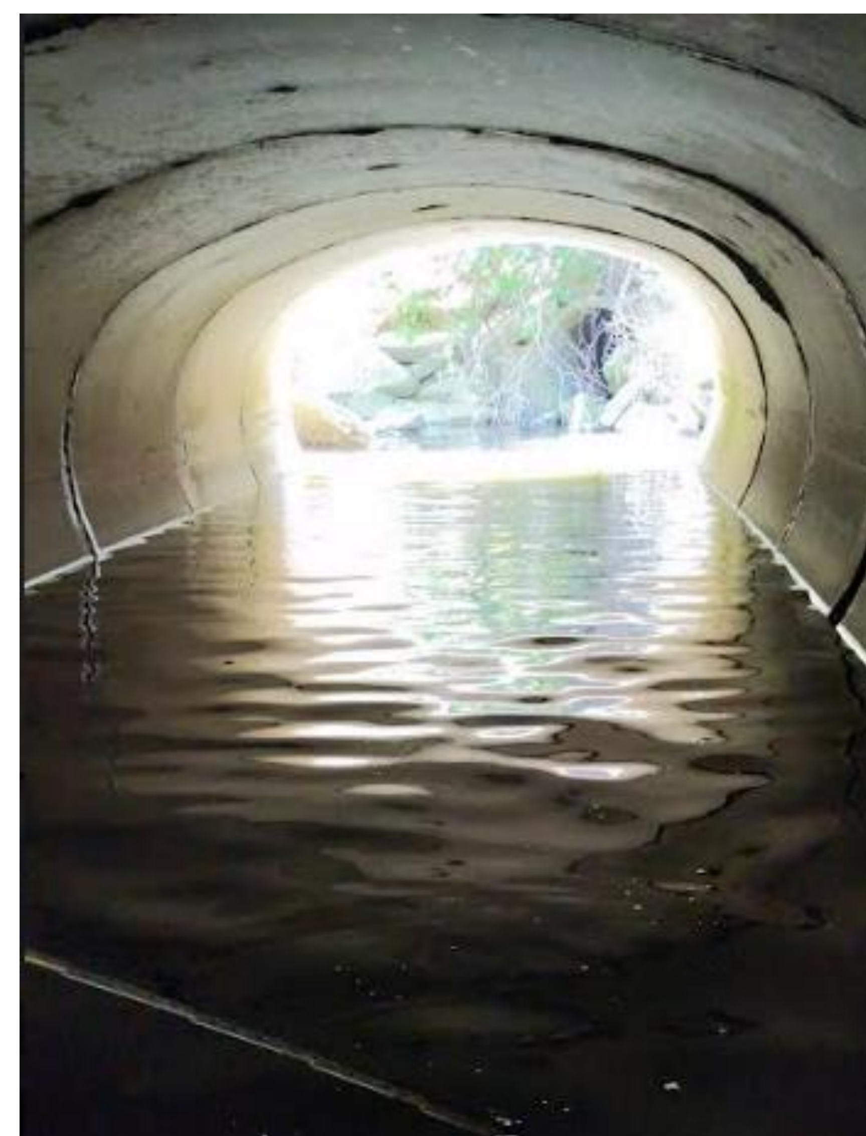
Figure 3. Wading through a culvert
