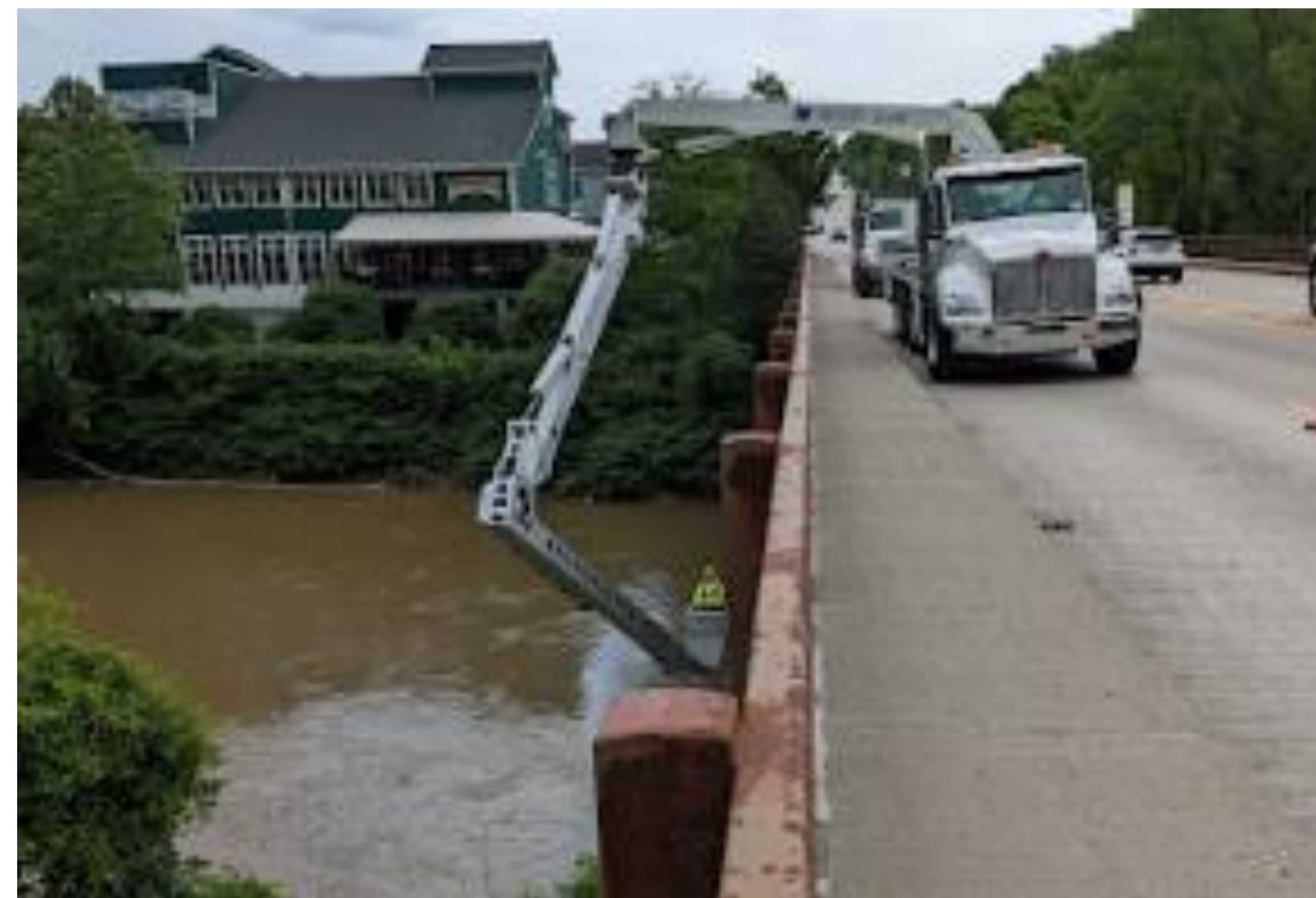
Figure 2. ODOT Snooper helps get up close with hard to inspect areas
