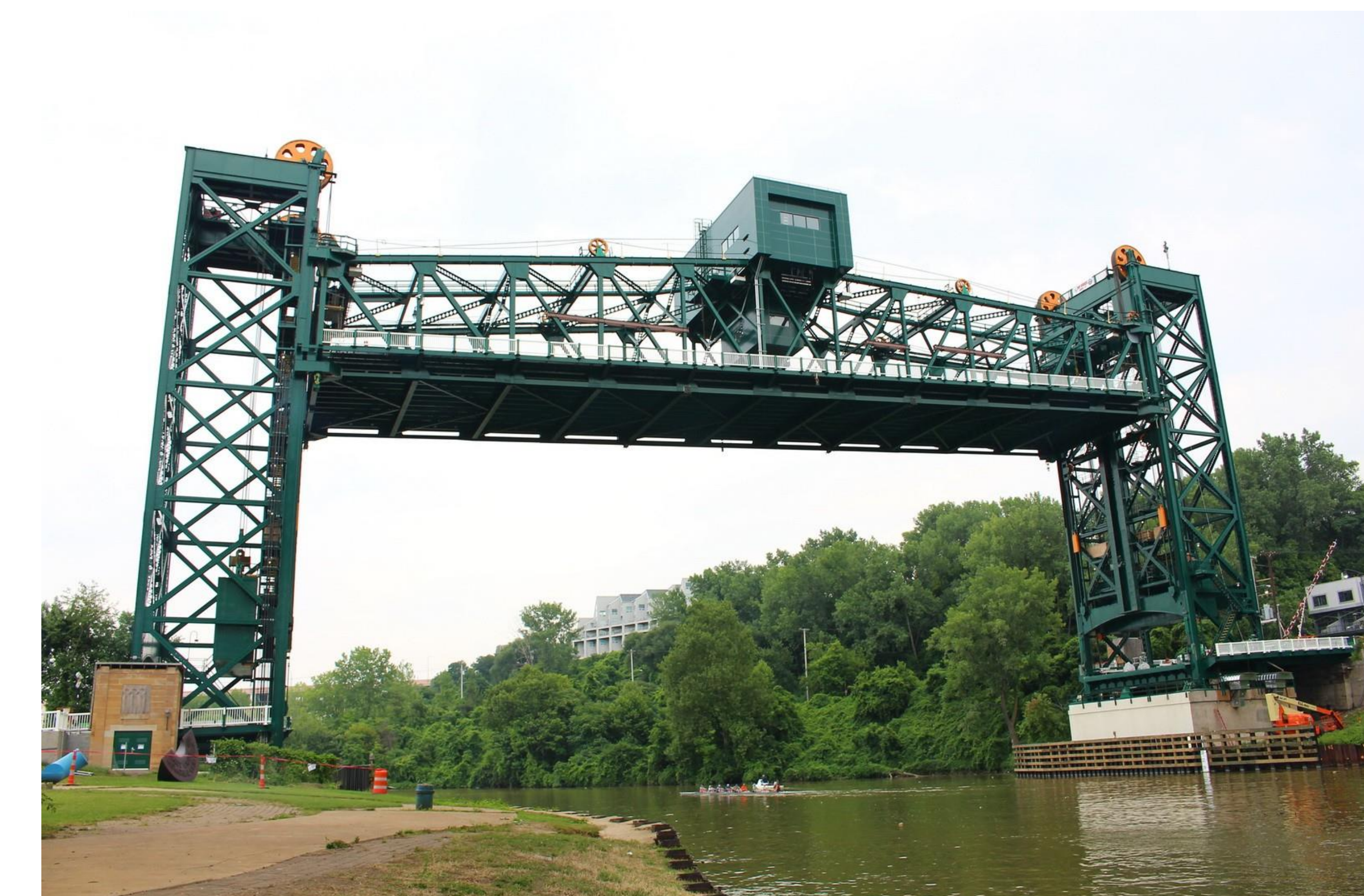
Figure 4. Columbia Road Lift Bridge
